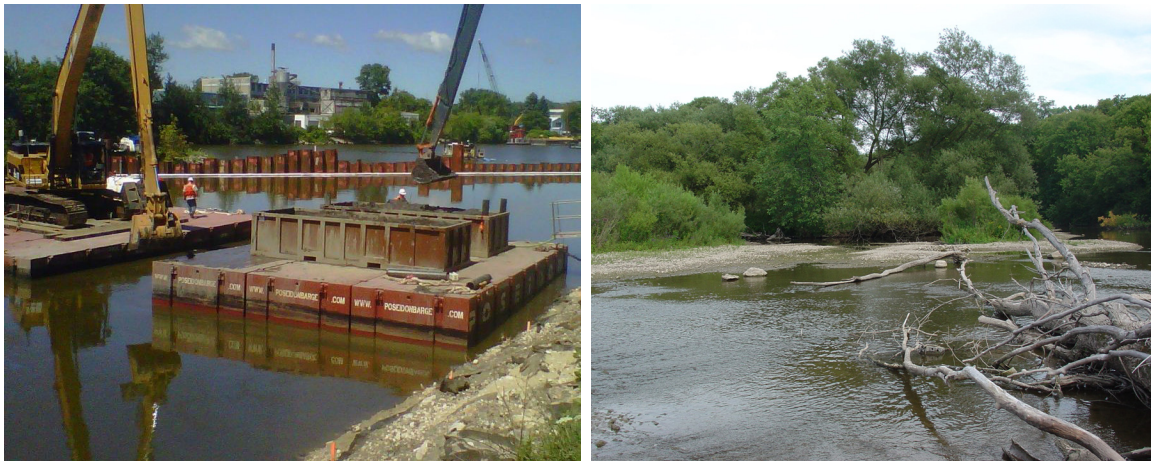
Figure 1. Toxic Sediment Removal (left) and Restored Habitat (right) along the Sheboygan River
